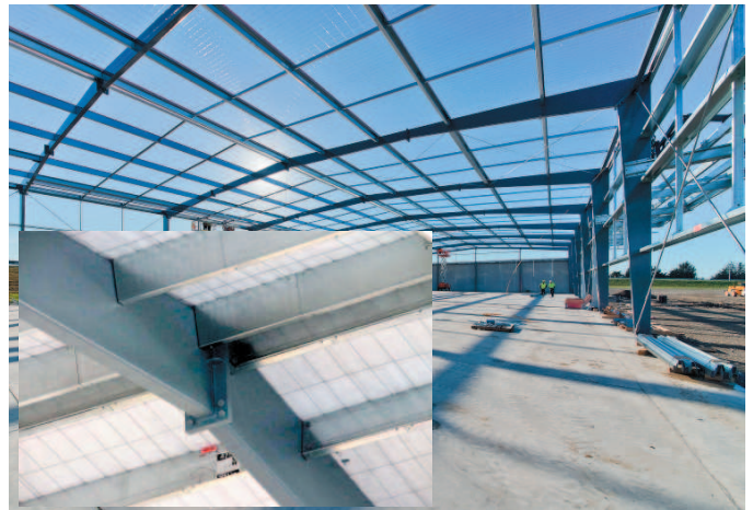
Steel construction innovation: HERA members Donovan Group and Steltech Structural's new Nested Tapered Box Beam solution for portal frames
