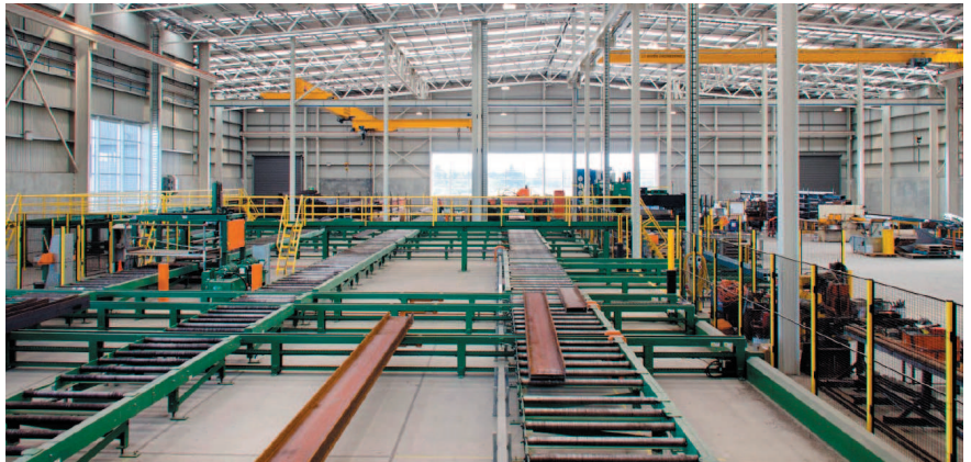
HERA member Calder Stewart Steel's innovative award-winning new structural steel fabrication facilities in Christchurch
