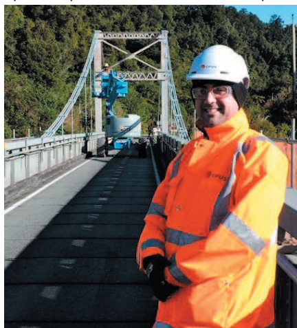
Former HERA Structural Engineer Raed El Sarraf now at HERA member Opus Consultants oversees the first use of the Ternmarst corrosion protection coating on a suspension bridge in the rugged west coast of New Zealand
