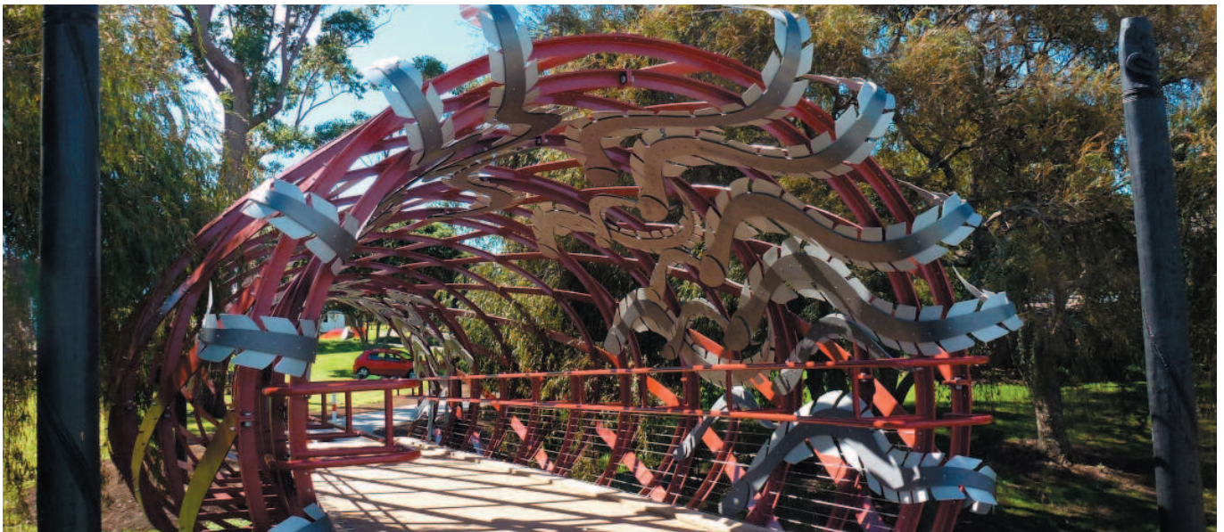
Eel Trap footbridge in Mt Roskill Auckland designed and fabricated by HERA members Beca and Eastbridge respectively
