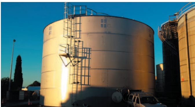
A technical first with new more cost-effective material: HERA member Acme Engineering's lean duplex stainless steel tank
